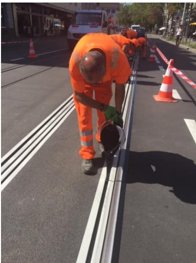
Picture 2: Application of Sikaflex-406 KC directly out of the pail
