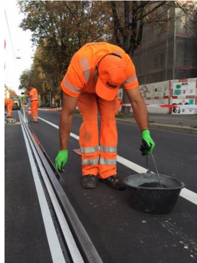
Picture 3: Broadcasting of Sikaflex-406 KC with quartz sand
